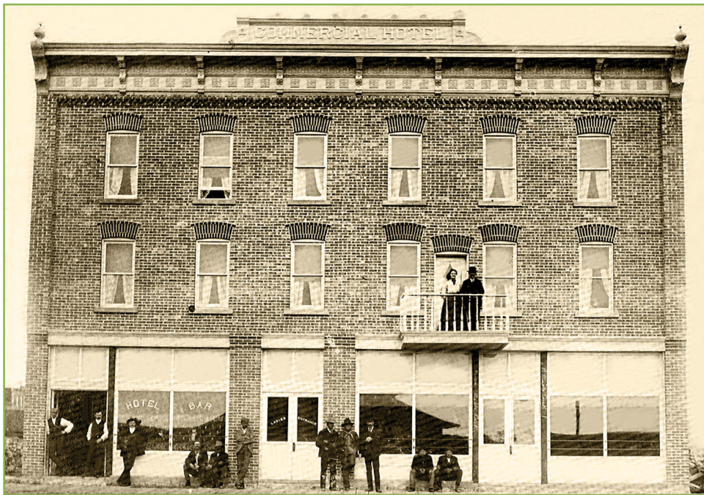
The 3-storey brick addition built by J.H. Fleming in 1906. The original wooden building was moved to the back of the lot forming the hotel's annex. It was demolished in 1940. After continued devastating floods, the brick structure was restored in 2014; it continued business as a hotel and restaurant until 2017.
